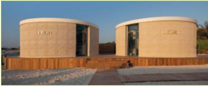
On Dubai's Jumeirah beach stands a unique Dior installation composed of two circular modules, crafted from natural materials—combining clay, sand and raw fibres using an exceptional 3D printing system designed by WASP ©Wasp
